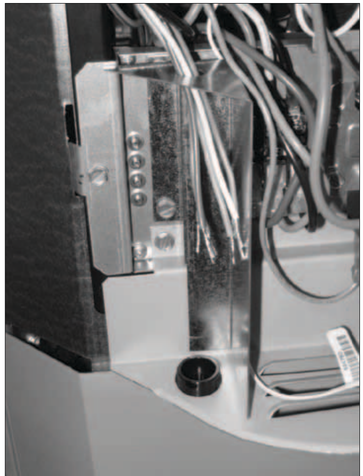
Figure 6. Low Voltage Compartment for Control Wiring
