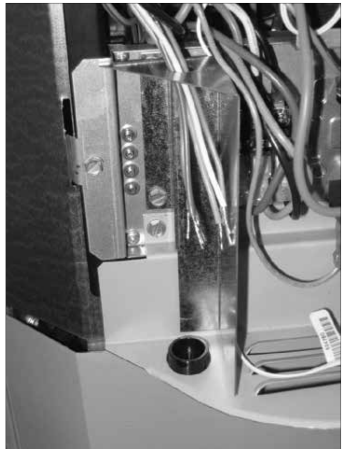
Figure 6. Low Voltage Compartment for Control Wiring
