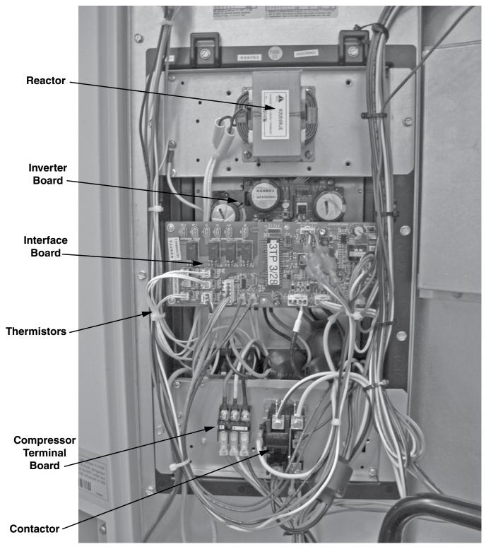
\* 5 Ton inverter assembly has additional components: Contactor, PTCR, and Fan Terminal Block
