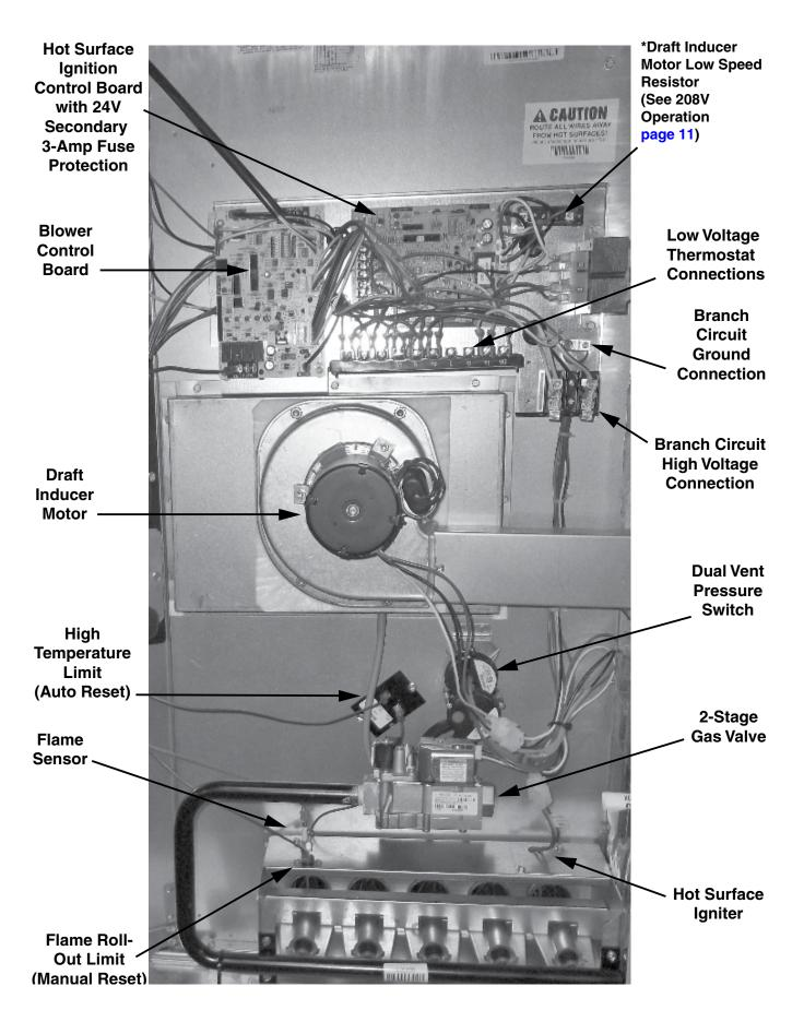
Figure 16. R6GI Typical Heat Exchanger Assembly
