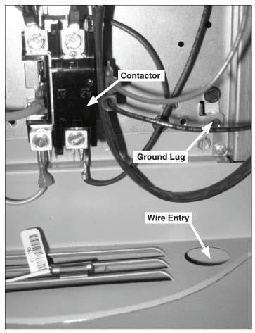
Figure 5. Power Wiring Terminals
