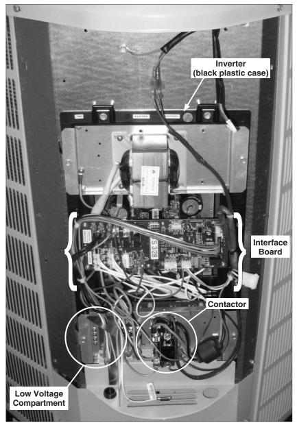
Figure 4. Heat Pump Control Panel (Cover Removed)
