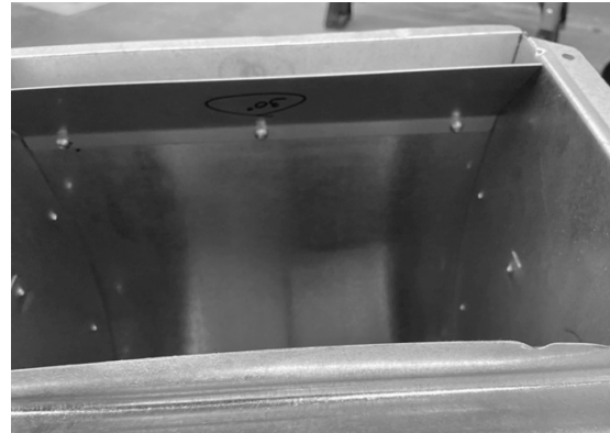
Figure 10. Installed Air Baffle, View 1
