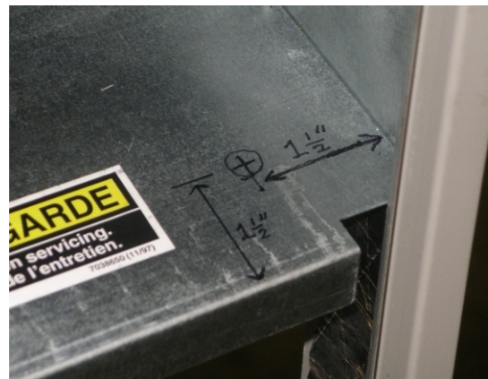
GAS HEAT MIXED AIR- SENSOR LOCATION
