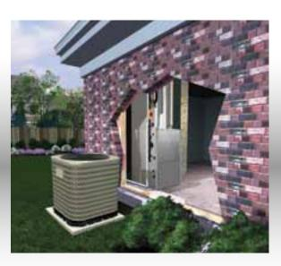
To qualify for an ENERGY STAR rating, split system air conditioners and heat pumps must have a Seasonal Energy Efficiency Ratio (SEER) rating of 15.0 or higher and an Energy Efficiency Ratio (EER) of 12.5 or higher. Split system heat pumps are also rated by a Heating Seasonal Performance Factor (HSPF) and must have a rating of 8.5 or higher.
