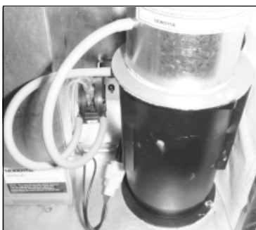
Picture 15. Combustion Air Blower
