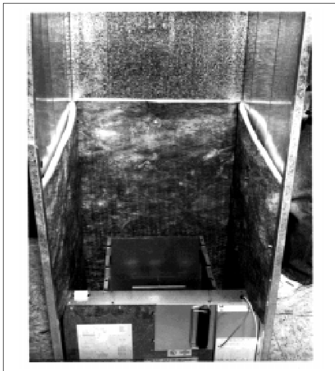
Figure 2. Evcon/Coleman furnace with insulation installed.
