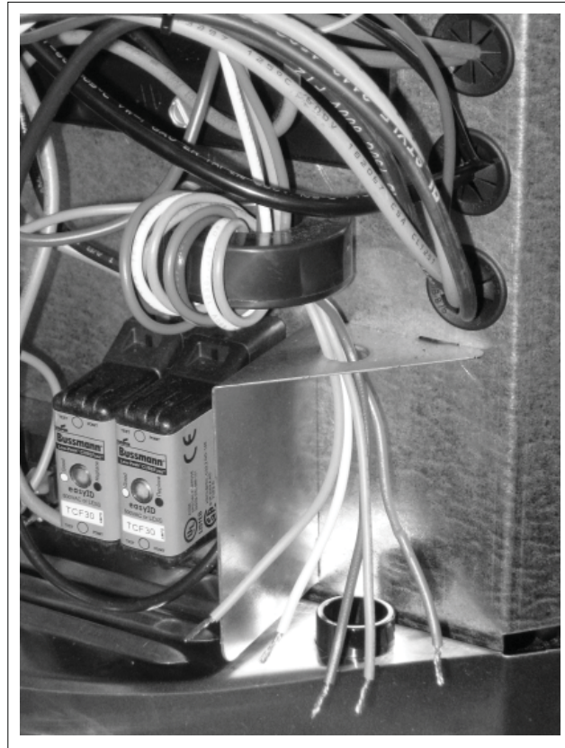
Figure 5. Low Voltage Compartment Control Wiring Connections
