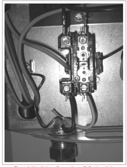
Figure 2. Line Voltage Connections, iQ Outdoor Unit
