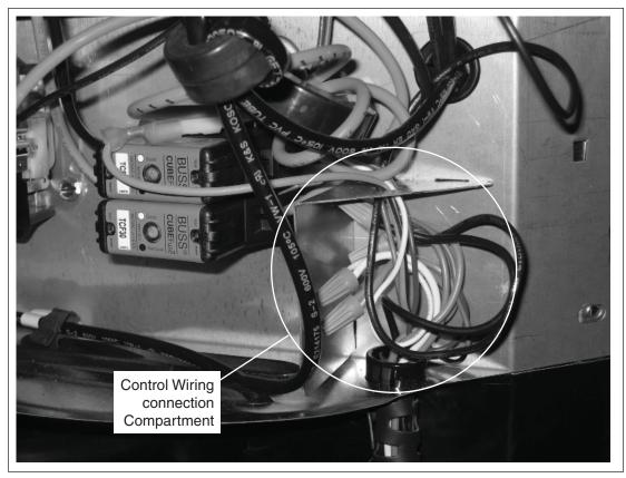
Figure 5. Control Wiring Connections, iQ Outdoor Unit (Air Conditioner Shown)
