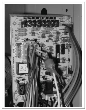
Figure 19. Two Stage G7 Furnace Board
