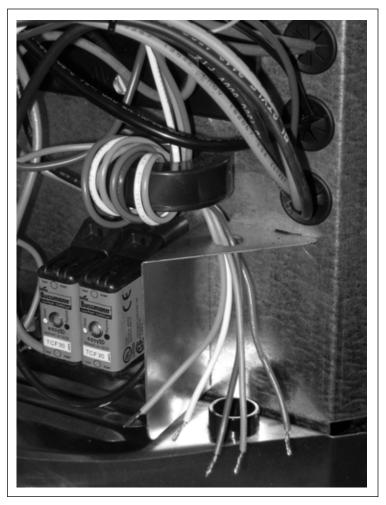
Figure 5. Low Voltage Control Wiring Compartment
