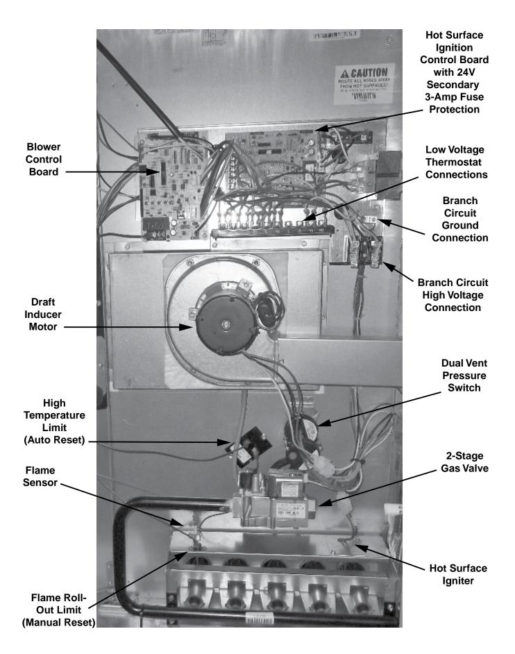
Figure 16. R6GI Typical Heat Exchanger Assembly
