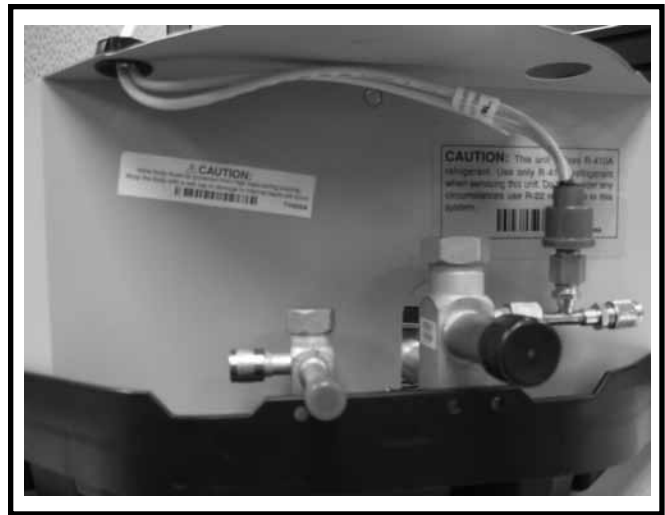
Figure 2. Wire Leads Through Grommet
