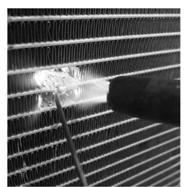
Figure 6. Brazing the Leak
