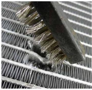
Figure 5. Micro-Channel Preparation
