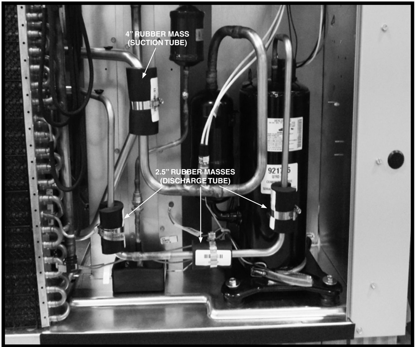
Figure 1. Anti Vibration Mass Locations
