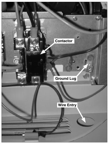
**Figure 3. Power Wiring Terminals**
