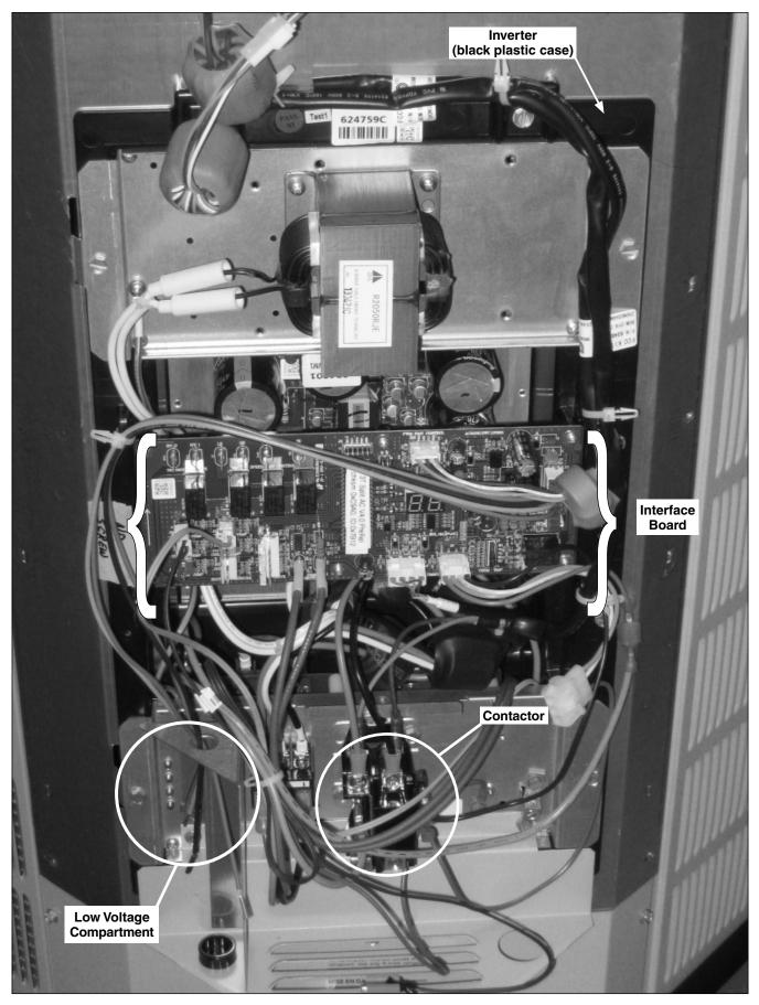
Figure 2. Air Conditioner Control Panel (Cover Removed)
